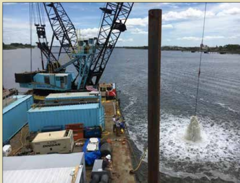
Airlift Dredging to clear area around the East Casemate.
