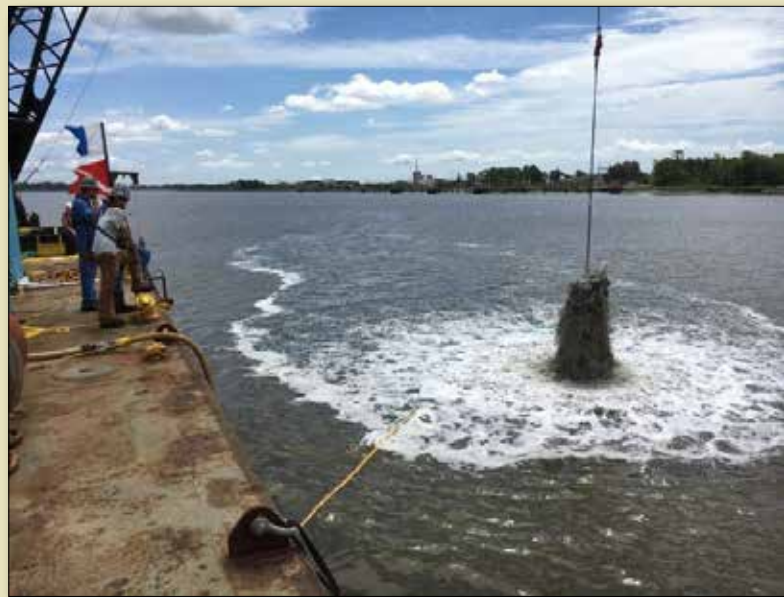
Airlift Dredging to clear area around the East Casemate.
