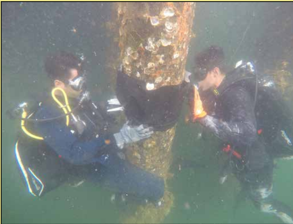
U.S. Navy and Army Divers participate in two weeks of pier repair events as part of a Joint Capability Technology Demonstration (JCTD) Event. This joint diving event is designed to provide our U.S. Diving and Engineering Teams with improved processes and technology to repair damaged port facilities due to natural disaster or kinetic effects. (Photo from PACOM JCTD Event Lead)
