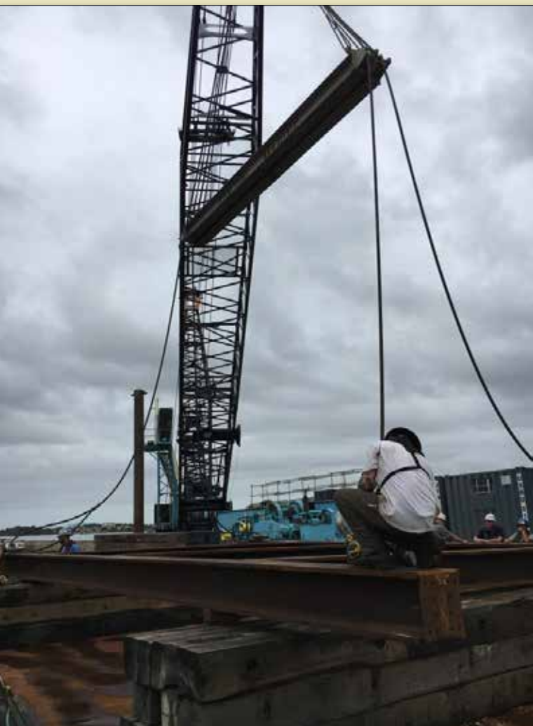
Shackling in the Lifting Frame and positioning for recovery of the East Casemate.
