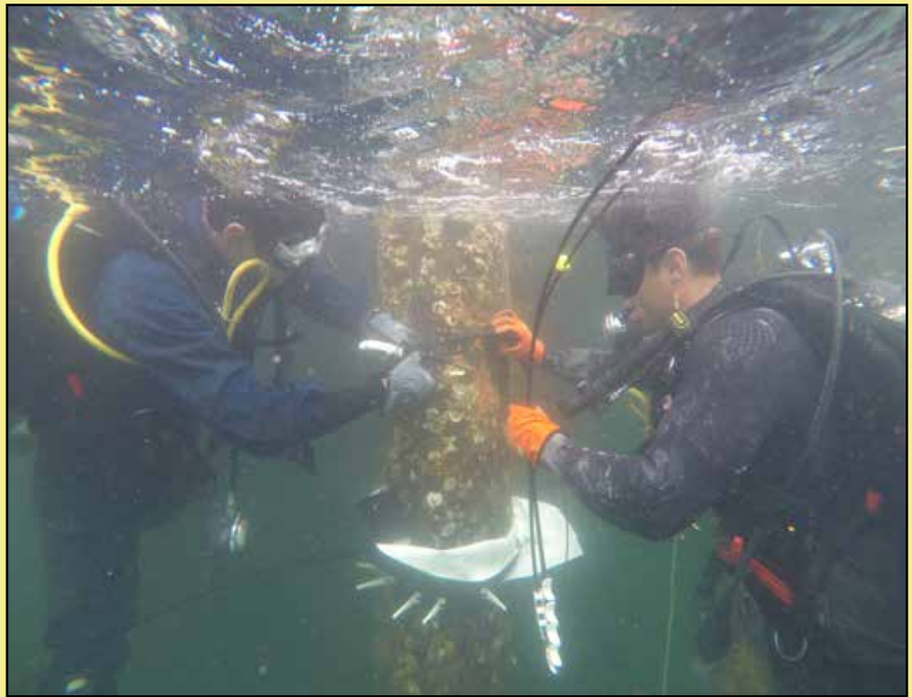
U.S. Divers prepare underwater pier piles for repair as part of a Joint Capability Technology Demonstration (JCTD). The event focused on improving our U.S. Army and Navy Diving and Engineering capabilities to rapidly repair ports that may have been damaged by natural disasters or in response to enemy kinetic action. (Photo from PACOM JCTD Event Lead)
