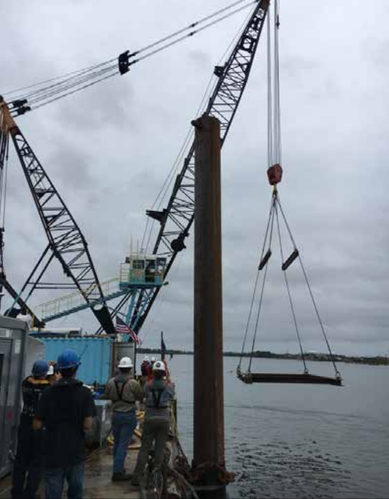
Shackling in the Lifting Frame and positioning for recovery of the East Casemate.
